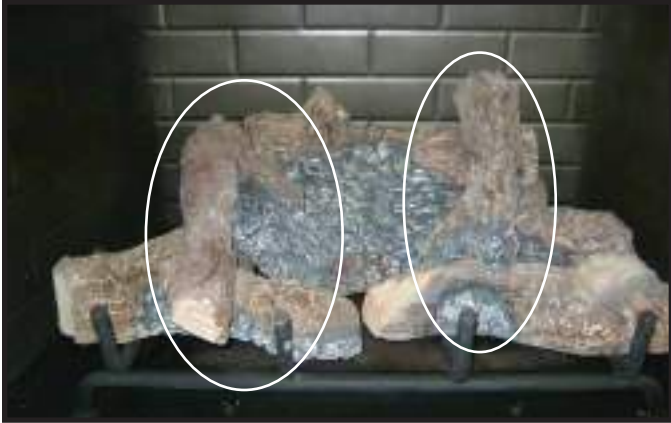
Figure 3.2 Remove Top Two Logs
