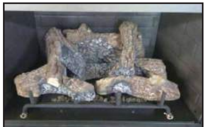
Figure 4. Left and Right Log in Proper Position
