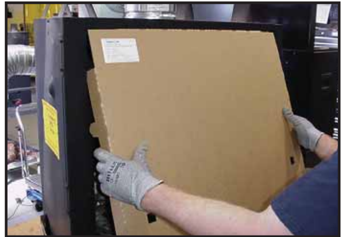
Figure 13.8 Installation of Splatter Guard
