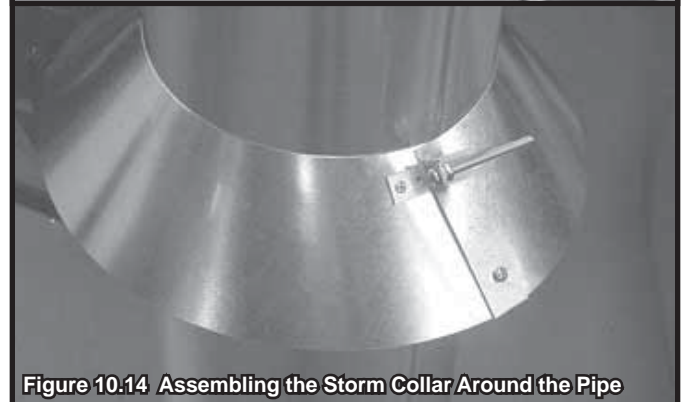
Figure 10.13 Assembling the Storm Collar
