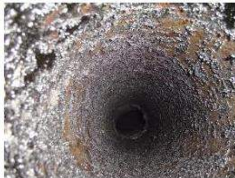
Flue before chimney sweeping
