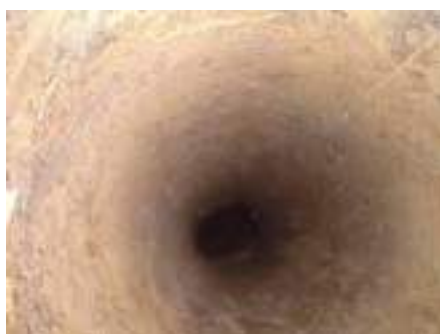
Flue after chimney sweeping
